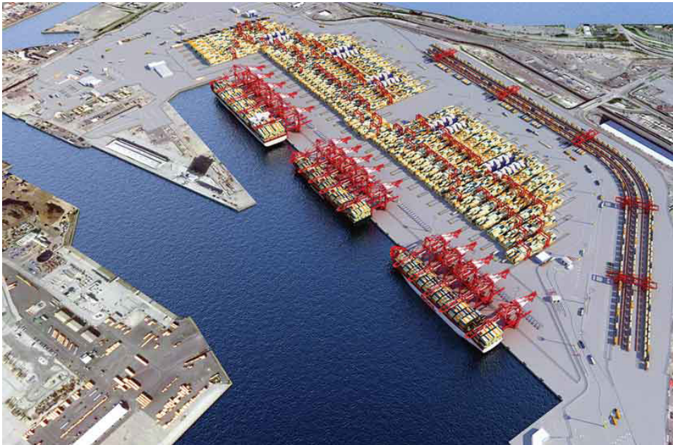
A nearly complete massive redevelopment program at the Port of Long Beach has created a fully automated terminal that includes automated vehicles. RENDERING COURTESY OF POLB
